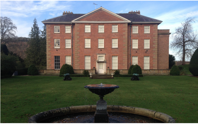
Brampton Bryan Hall, near Leintwardine, in South Shropshire. Graham's team was responsible for all the electrical services for this Georgian mansion
